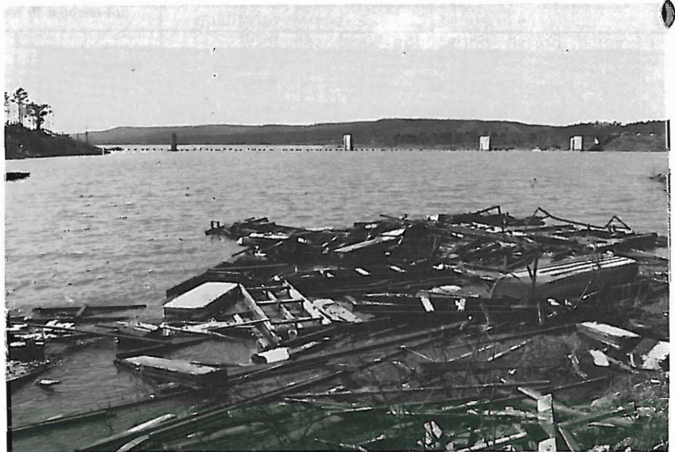
Debris from a destroyed boat dock clutters the lake front near the remains of the Highway 16 bridge. View is looking toward the west.
