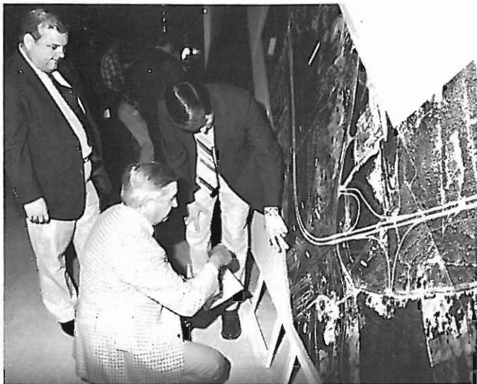
Roadway Design Engineer Bob Walters, right, explains features of the North Belt Freeway to State Representative Dave Roberts, center, and Highway Commissioner Raymond Pritchett.
